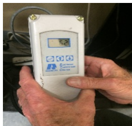
Control unit for chiller
